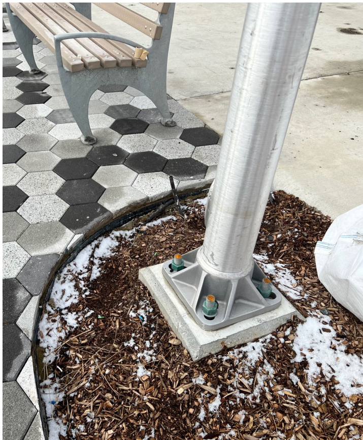
Poor Spacing Ensure enough space around pole for planting
