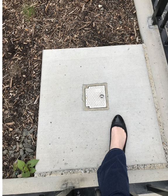
This concrete pad for ground hydrant in planting is too large though its location abutting the curb is in a good, unobtrusive location
