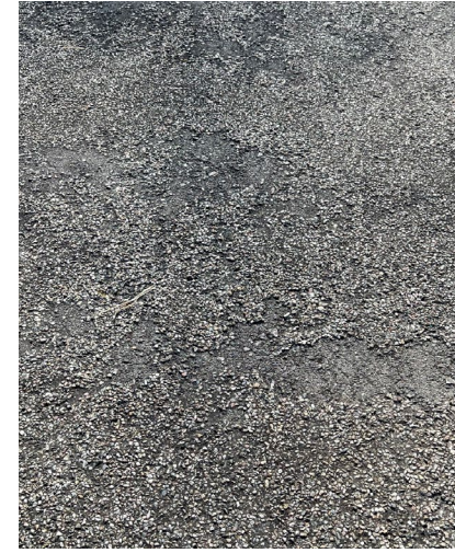
Asphalt with aggregate rolled into top course
