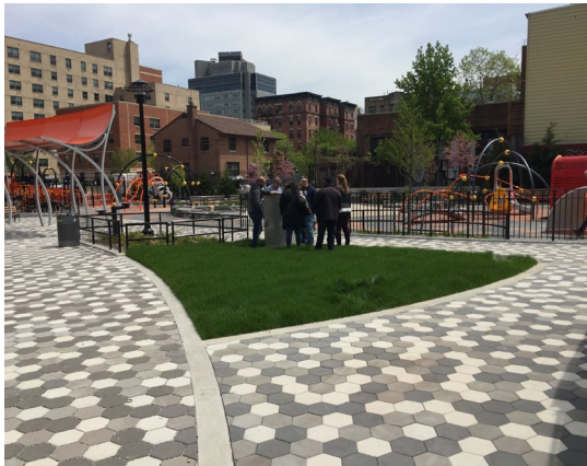
Concrete curbs binding concrete pavers
