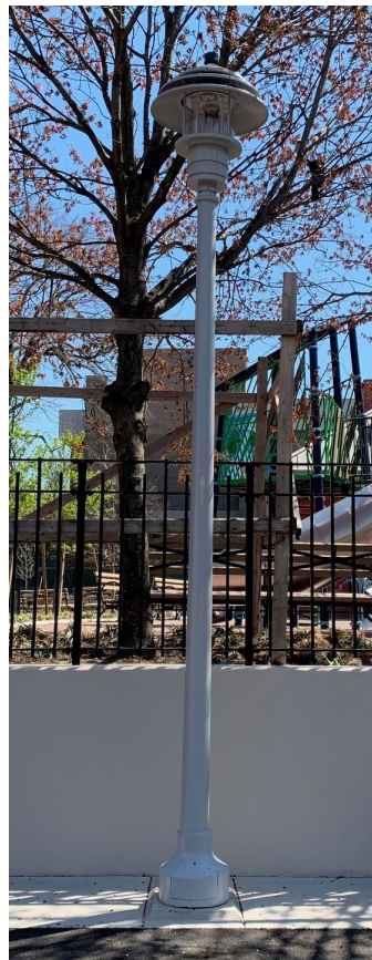
Wrong Color Ensure proper color in shop drawings and construction Flushing Meadows Luminaire and Pole
