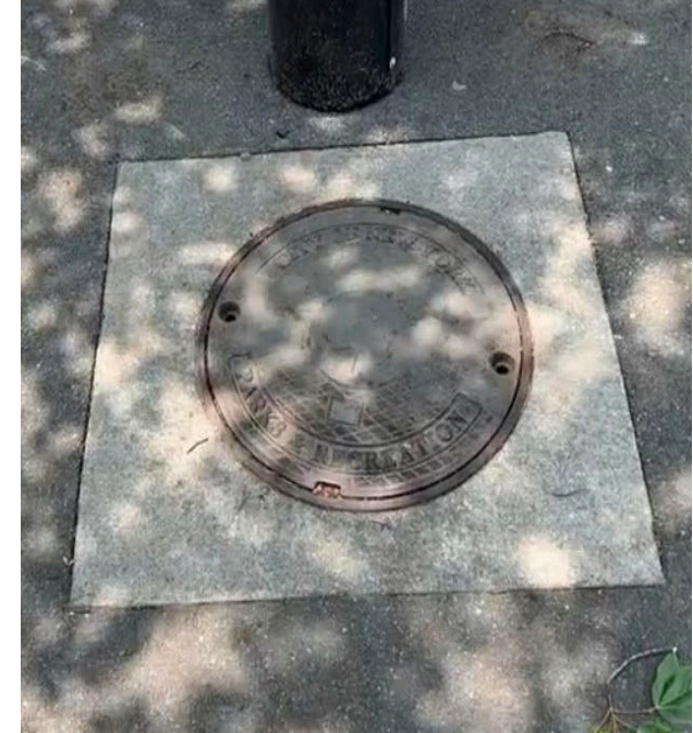
Avoid unnecessary concrete pads (and small hard to roll asphalt areas)
