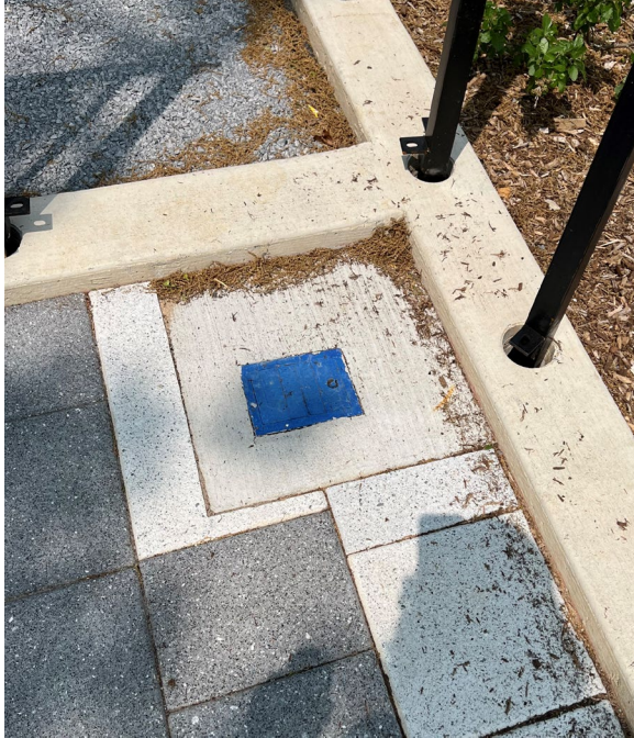
Concrete pad is not required for ground hydrant when in concrete or in asphalt pavers
